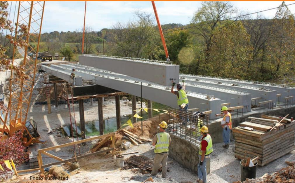
The *closed loop structural tied arch system* housed in a composite shell will extend the expected service life to 100 years.
